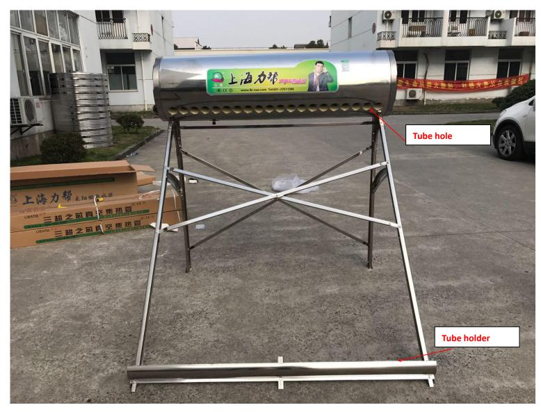
Caution: Tube hole in the tank must align to tube holder. Otherwise, 1, tank maybe leakage. 2, Vacuum tubes will be crushed.
