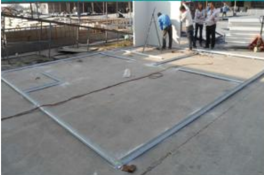
U ground and lock channel
